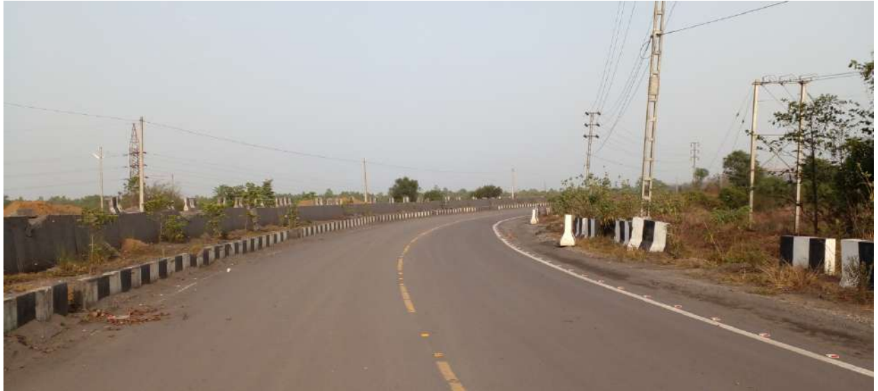
Black topped road of length 2700m and width 8.5m from Bankbahal towards Raigarh for LMV
